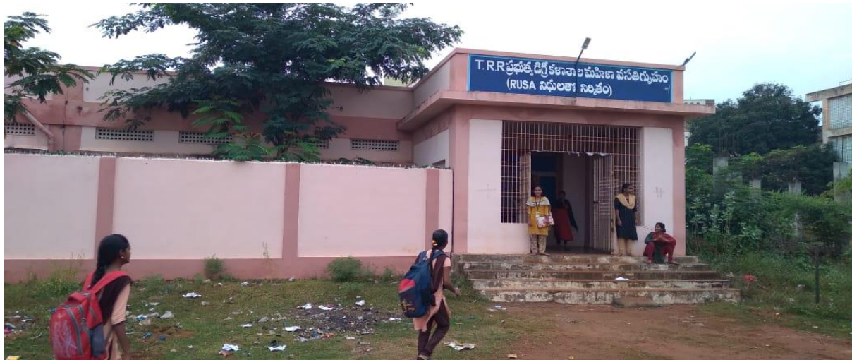
The Social welfare Girls hostel shifted to new building which was constructed under RUSA funds in college premises.
