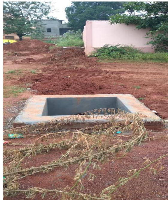
Girls hostel drainage problem has been resolved by construction of underground drainage system
